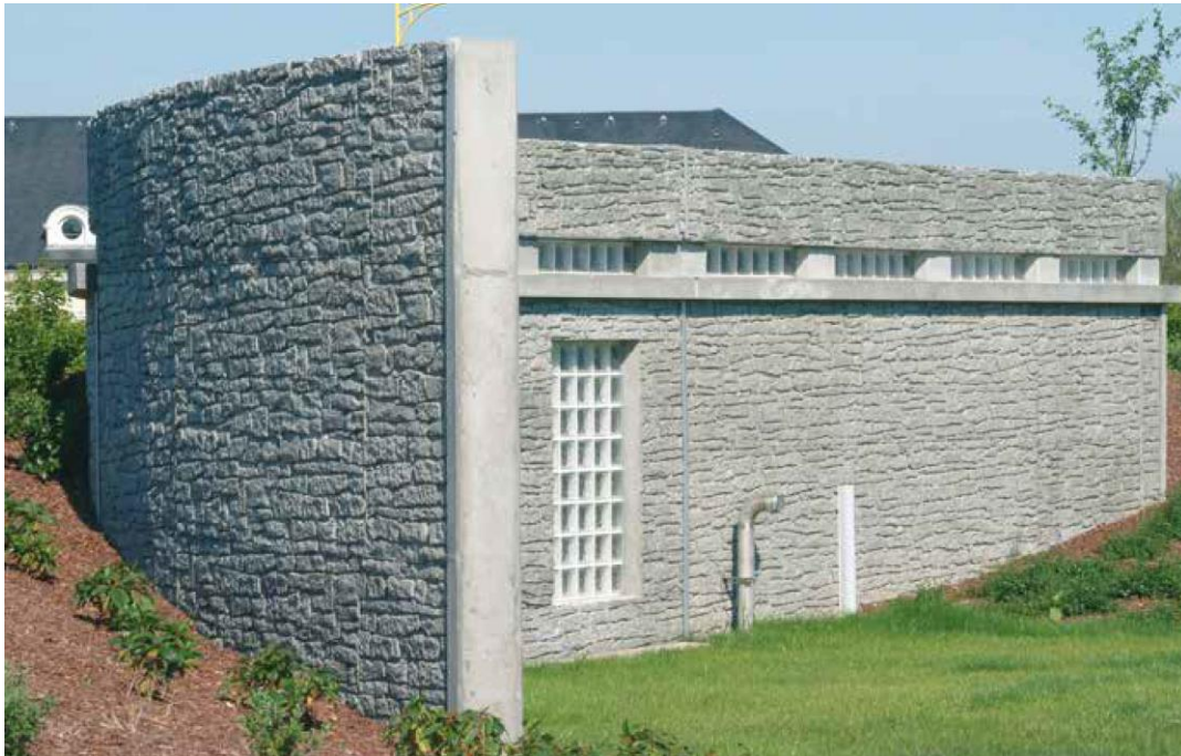
Figure 1-8 - Insitex formwork liner feature finish
