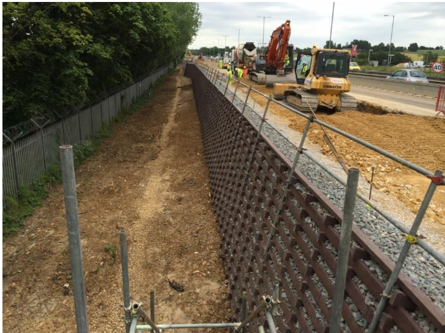
Figure 1-7 - Eco-Crib Retaining Wall
