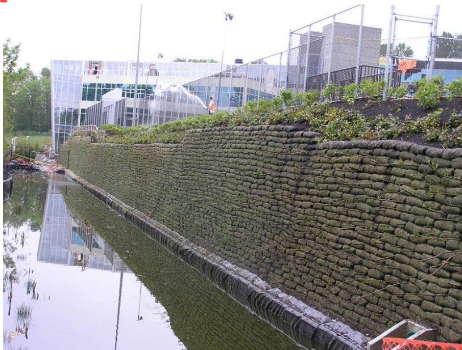
Figure 1-9 – Flex-MSE – live staked and hydroseeded
